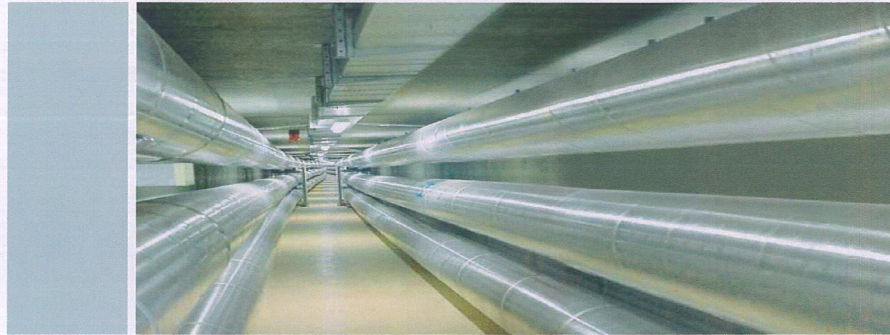
300 kV GIL system (operating voltage 220 kV) for Palexpo in Geneva (Switzerland), commissioned in 2001
