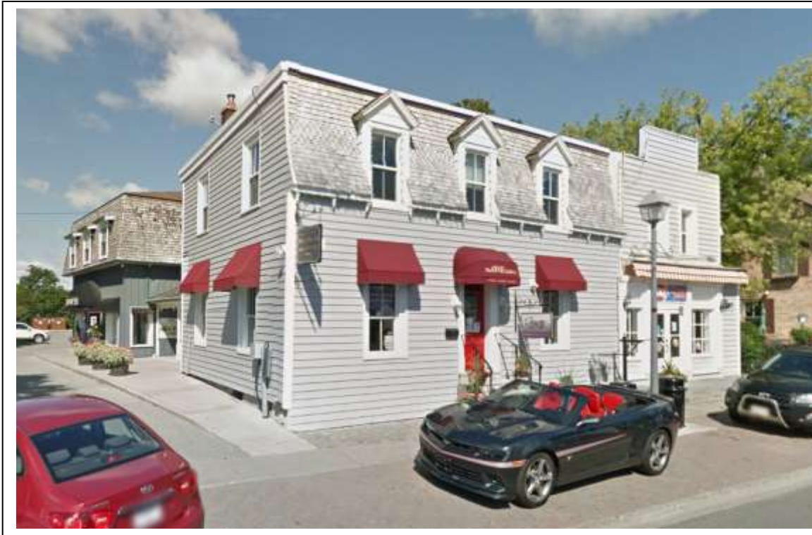
FIGURE 4 – Building with Work Completed
